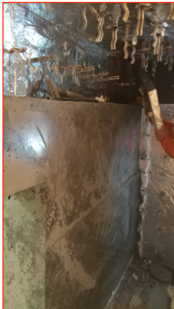
Installation of a High-Efficiency Refractory Lining (HERL)
