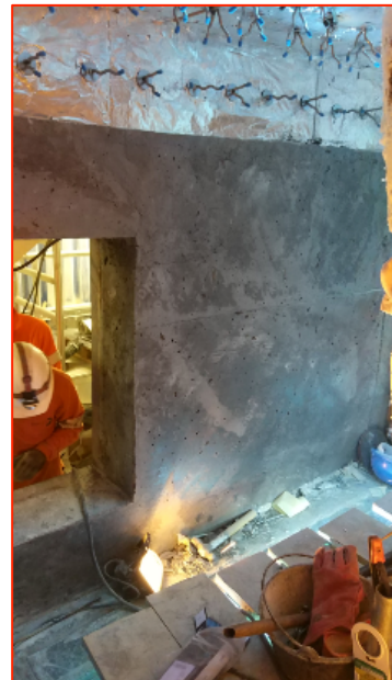
Installation of a High-Efficiency Refractory Lining (HERL)
