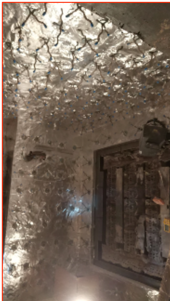
Installation of a High-Efficiency Refractory Lining (HERL)
